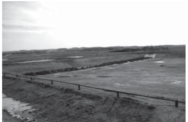
Leach pad construction
