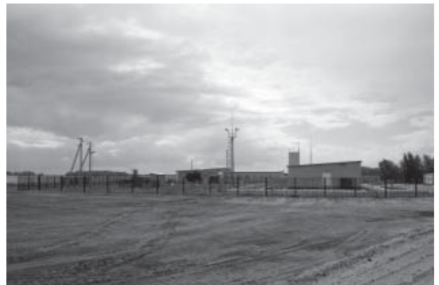
Camp, with facilities to house 110 people at Uzboy site
